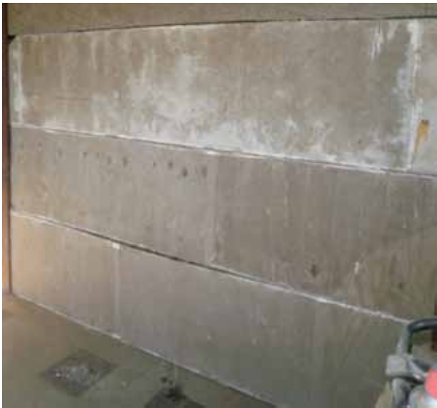
Figure 4. Precast geopolymer concrete wall (8 ft. x 11 ft.) designed to hold back 300 t of soil.
